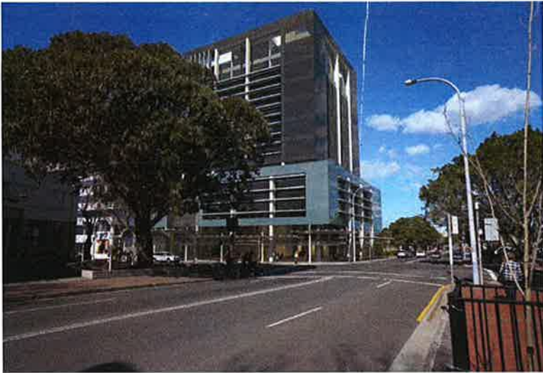
VIEW FROM NORTH
